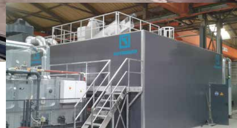
Noise reducing cabinet around the shotblast machine.
