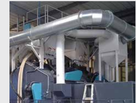
Optimal air filtration by highly effective exhaust plant.
