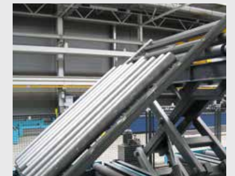
Special tilting devices to empty blasted pipes from abrasive.
