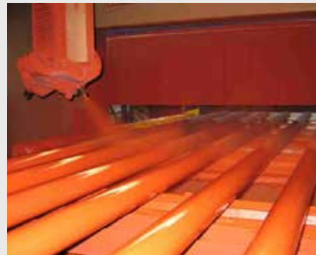
Simultaneous application from top and bottom side to achieve complete painting in a single movement.
